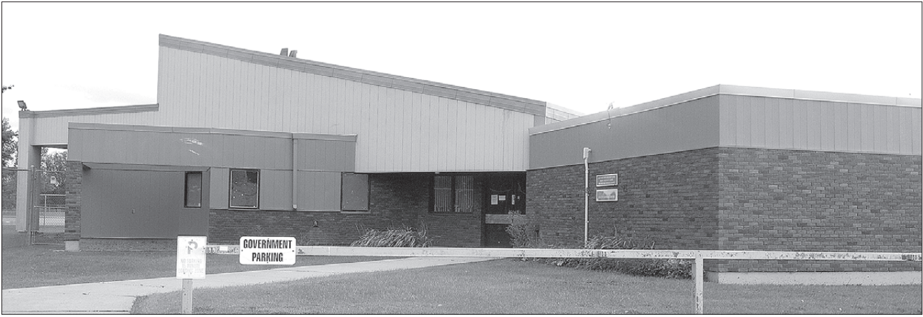
The High Prairie Youth Assessment Centre was damaged by fire in November 2023. Town of High Prairie Mayor Daniel Vandermeulen toured the building Aug. 7 and says the building was not extensively damaged.
